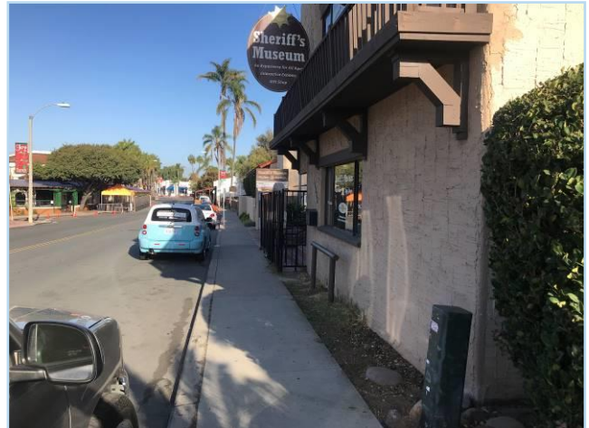
West elevation along San Diego Ave
